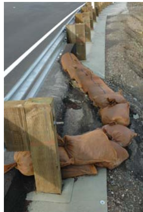
Figure 4. Sandbag berm.
