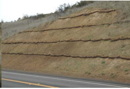
Figure 2. Mulch and wattles on steep road cut.
